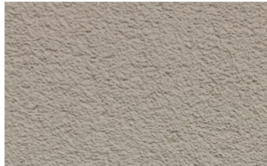
CLADDING* Dulux Pipe Clay
